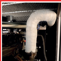
Exhaust pipes with exhaust heat wrap for high-performance and security
