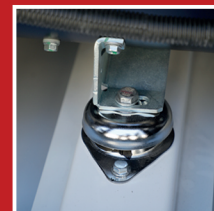
Anti-vibration pads attenuate the vibrations caused by the unit
