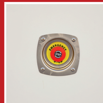
Emergency stop button It shuts down the generating set immediately
